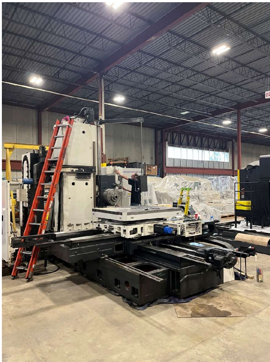
Installed Table and saddle
