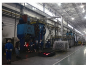
德阳东汽叶片CHK80kJ-CTK125kJ 2条模锻线 CHK80kJ-CTK125kJ vane forging lines in Deyang Dongfang Turbine Co.,Ltd (2 lines)
