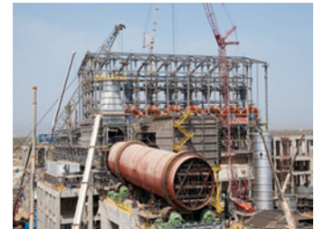
Structural steel manufacturing
