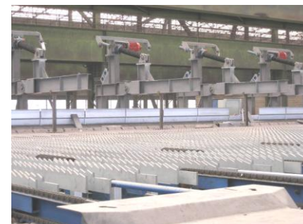
Working Level of Cooling Bed
