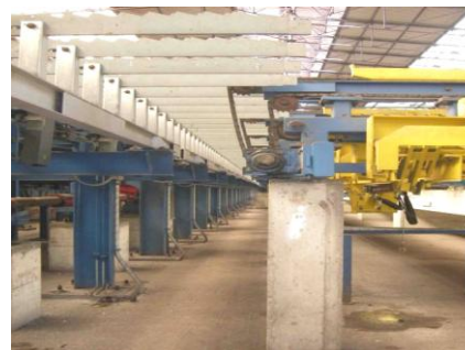
Foundation of Cooling Bed
