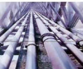
Thickness check of pressure pipelines
