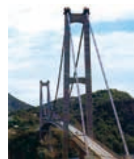
Routine maintenance of roads and bridges
