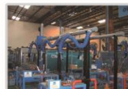
直线焊接专机除尘 Straight seam welding machine dust removal
