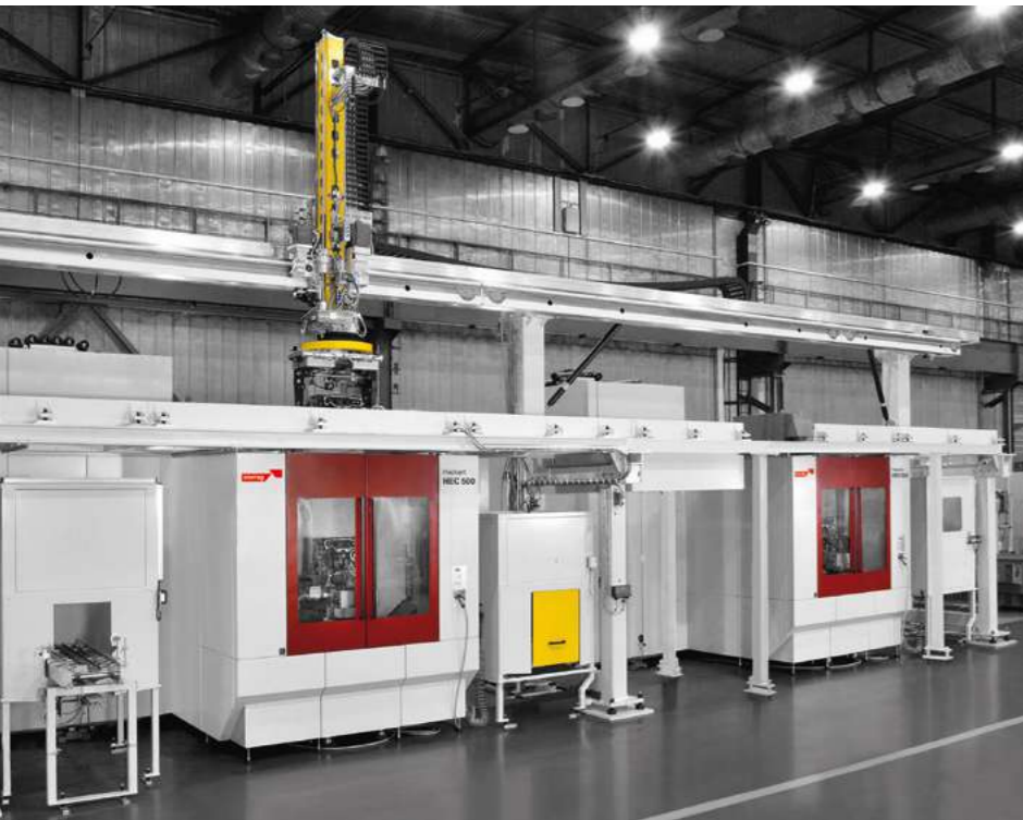
Production line with 3 machining centers Heckert HEC 500 Athletic and workpiece transfer by gantry robot for fully.
