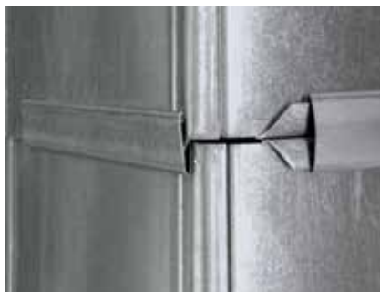
„S“ seam and drive cleat
