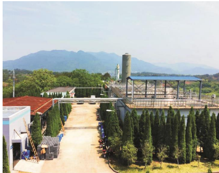
兰溪市黄店镇150吨每天垃圾渗滤液处理工程 150T/D Landfill Leachate Treatment Project in Lanxi City
