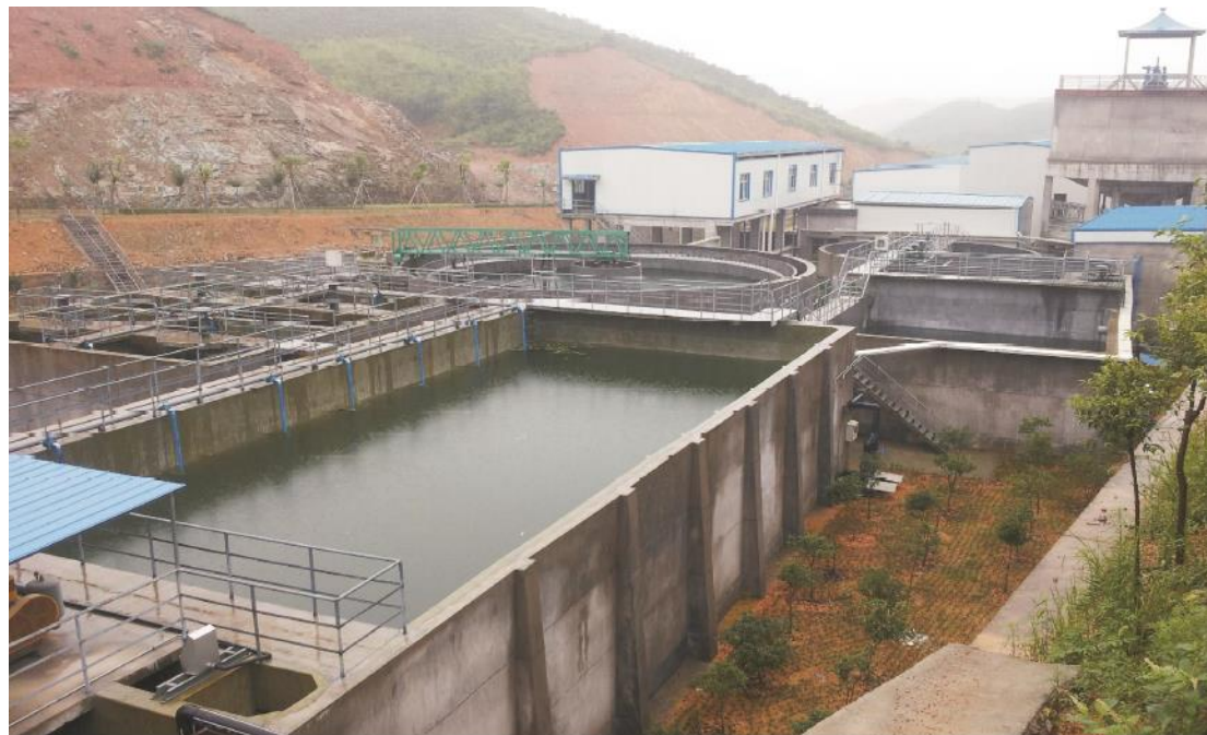
▲ 浙江豪美钒业有限公司3,000吨每天石煤提钒废水处理及900吨每天回用工程 3,000T/D Extracting Vanadium from Stone Coal Waste Water Treatment and 900T/D Water Recovery Project for Zhejiang Haomei Vanadium Industry Co., LTD
