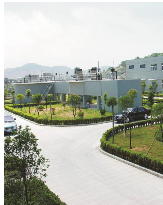
▲ 舟山定海40,000吨每天污水处理厂（一、二期）工艺设备 Process Equipment Supplying and Installation Project of Treatment Plant (Phase I, II) of Zhoushan Dinghai WWT
