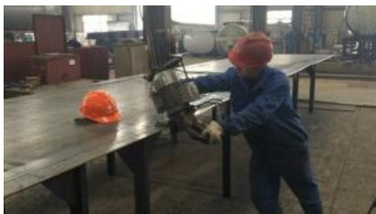
应用现场 ON-SITE PROCESS
